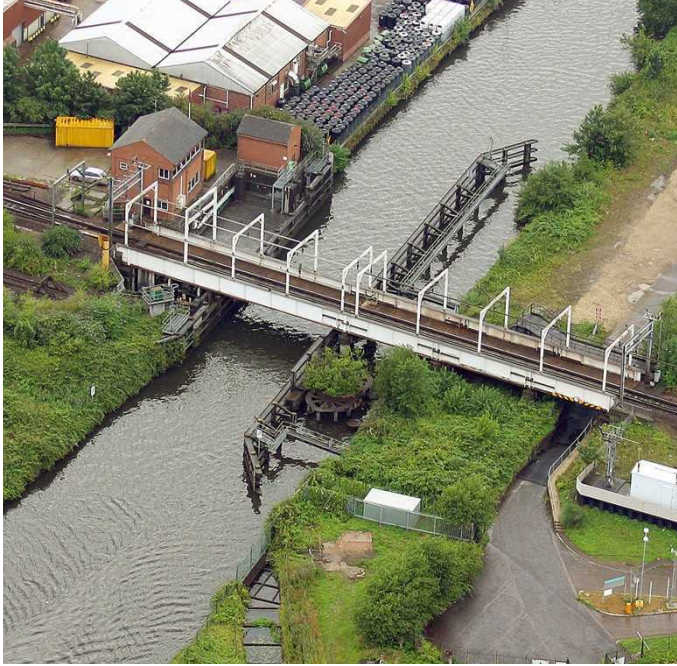
Trowse swing bridge – image courtesy of Mike Page – www.mike-page.co.uk
