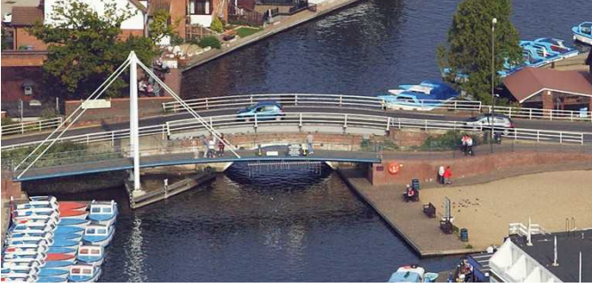
Wroxham road bridge – image courtesy of Mike Page – www.mike-page.co.uk
