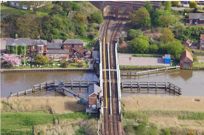
Reedham swing bridge – image courtesy of Mike Page – www.mike-page.co.uk
